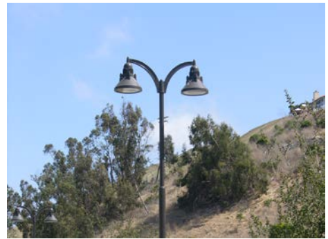
Figure 44. Hooded light fixture directs light downward.
