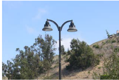
Figure 12. Hooded light fixture directs light downward.
