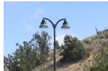
Figure 12. Hooded light fixture directs light downward.
