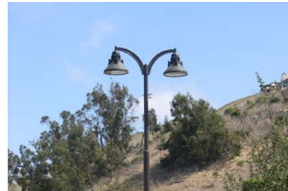
Figure 12. Hooded light fixture directs light downward.
