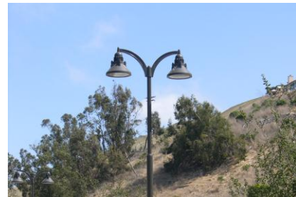
Figure 12. Hooded light fixture directs light downward.
