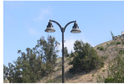
Figure 44. Hooded light fixture directs light downward.
