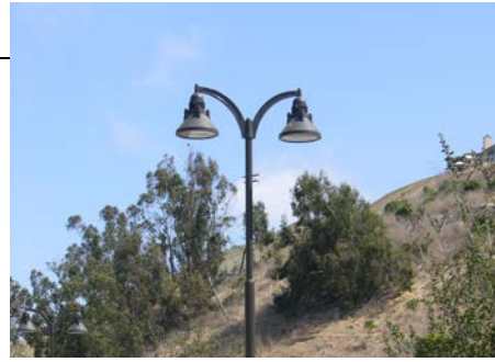
Figure 44. Hooded light fixture directs light downward.
