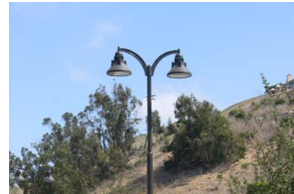
Figure 12. Hooded light fixture directs light downward.
