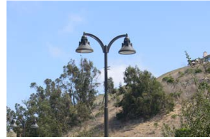
Figure 12. Hooded light fixture directs light downward.
