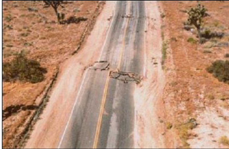
Figure 4-8: Surface Rupture
