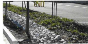
Figure 5-2. On-site storm water capture system.
